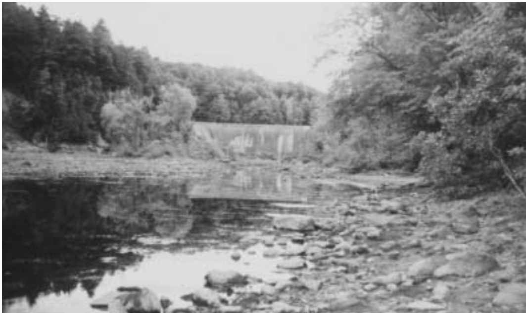
The Peterson Dam
