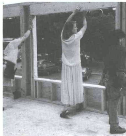
All VNRC staff hands were needed to frame this summer's addition.
