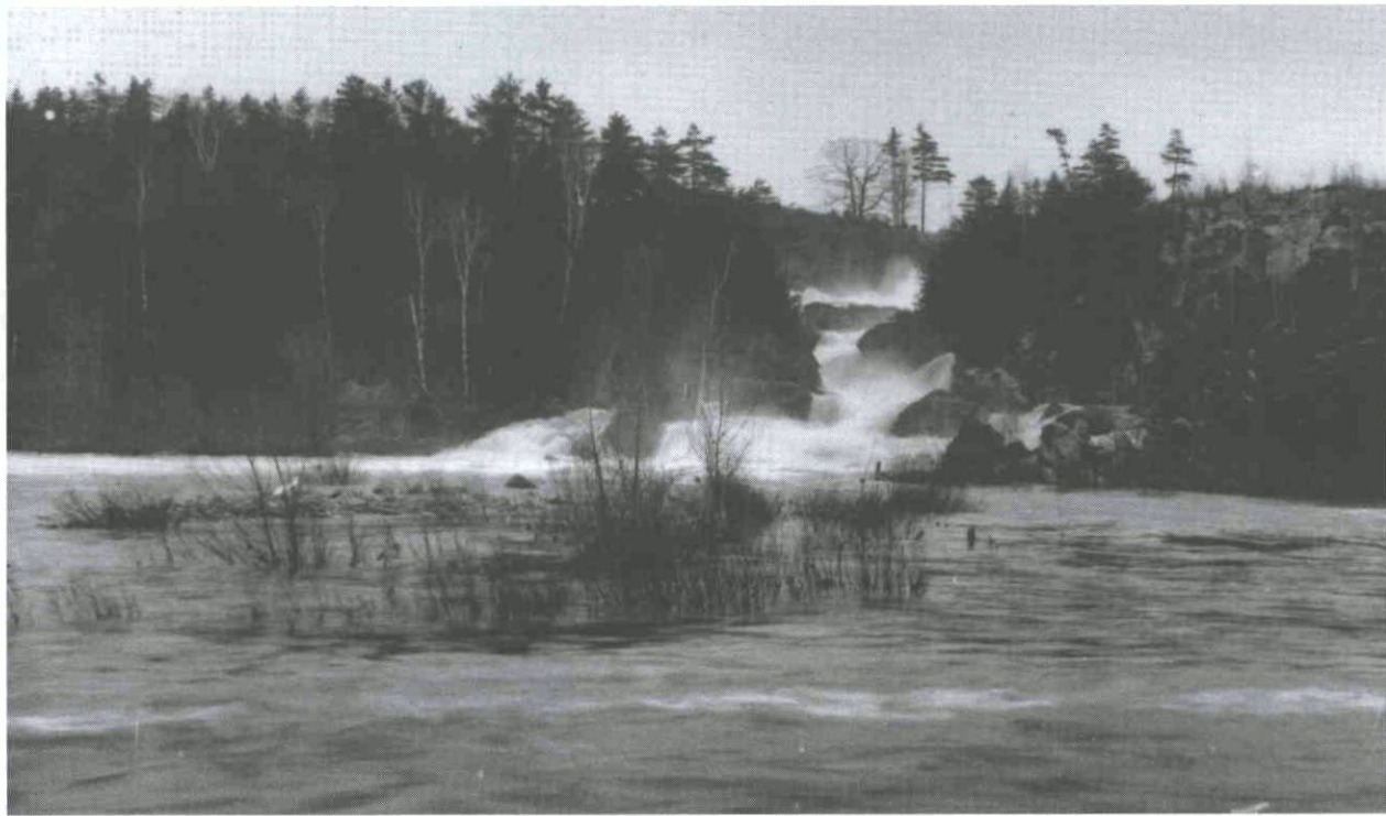
A free-flowing Lamoille River cascades over Milton Falls in 1909 before the waters were harnessed for hydropower.
