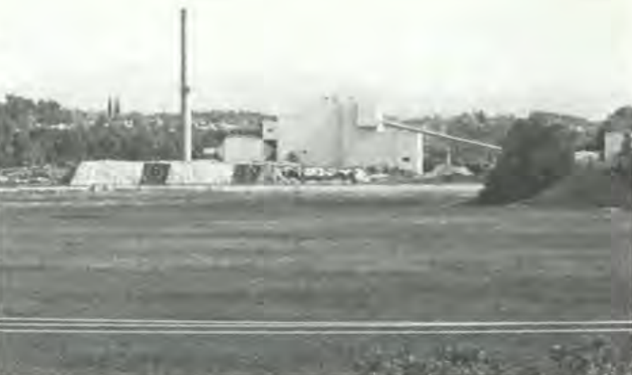
Above: The McNeil plant on Burlington's intervalle. Photo by Kathy Bond.
