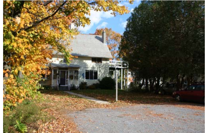
This building on Maple Street houses one apartment and two businesses.
