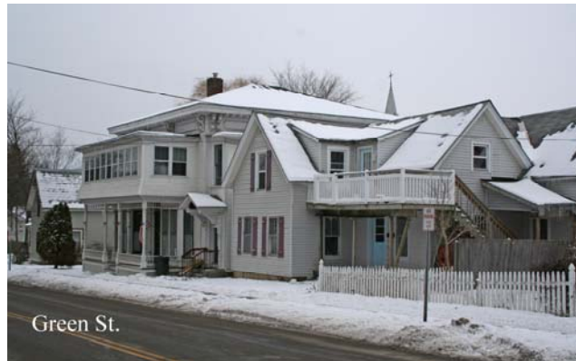
Three unit apartment building on Green Street.
