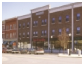
Infill building, Randolph, VT
