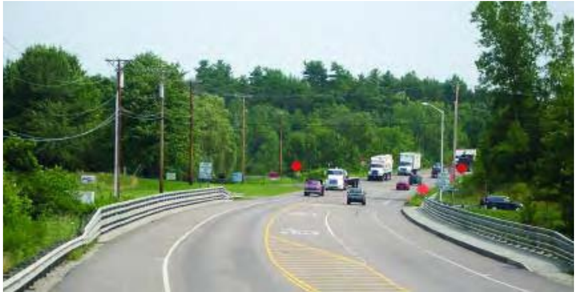
Figure 4.4: Compatibility of Bridge Design with Surroundings. Both of these recently constructed bridges are entries to historic villages. The dark railings, more decorative streetlights, and smaller scale of the bridge in the lower picture are sensitive to the historic village and create a more compatible gateway.
