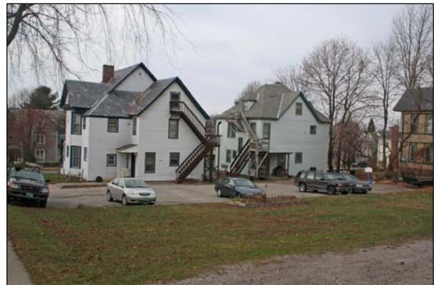
Parking area behind two 6-unit apartments on S. Union St.
