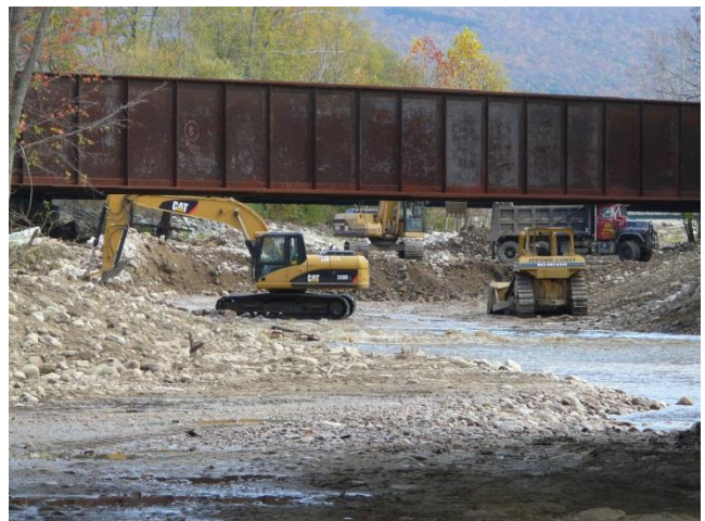
Dredging to open up Roaring Branch in Bennington
